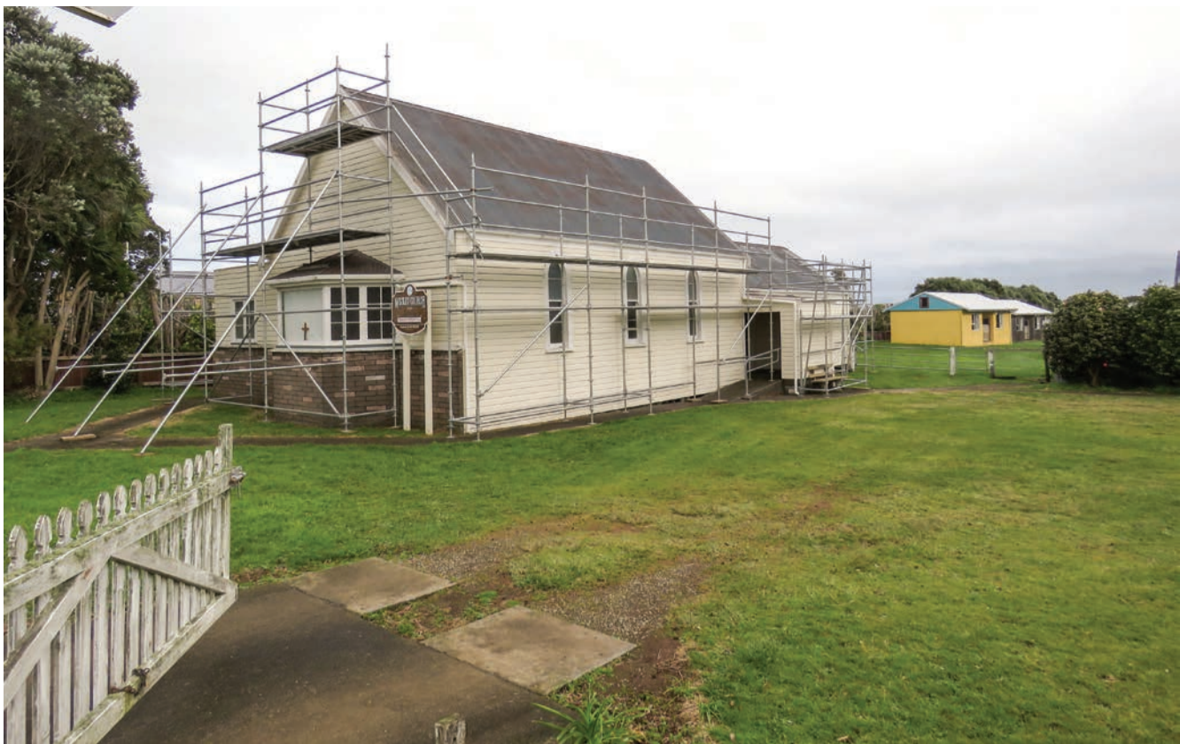
The historic Methodist Church in Rahotu about to be re-roofed.
